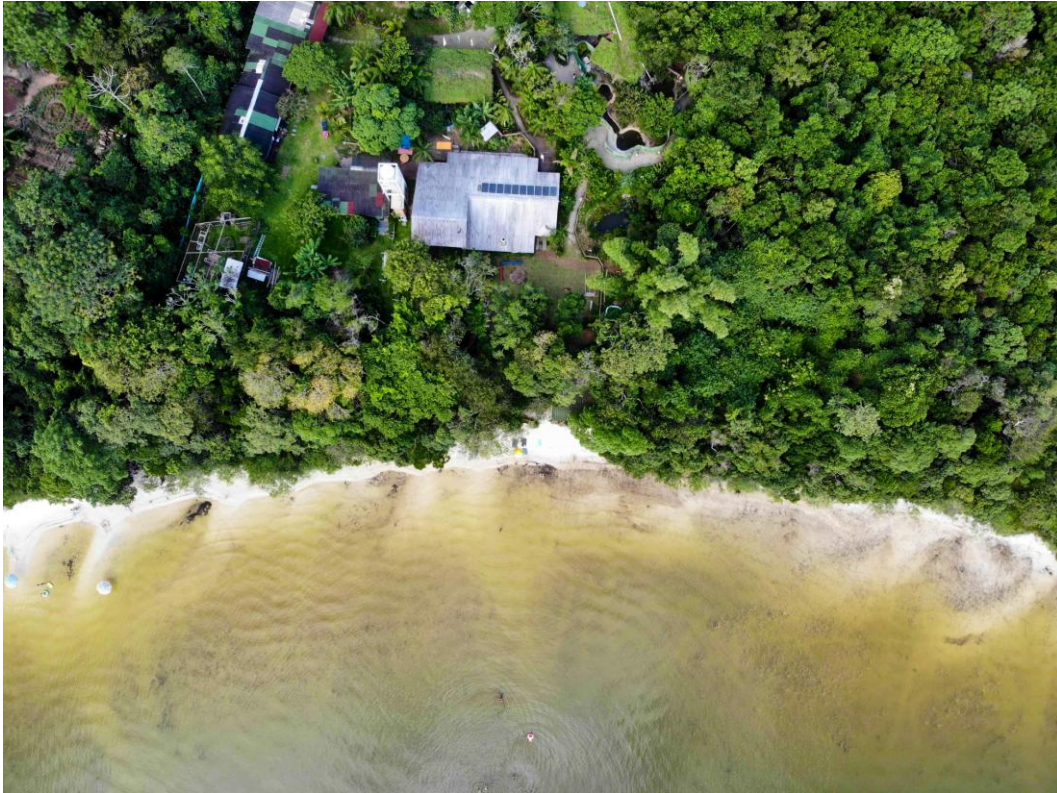
Figure 1. The Visitation Center (larger roof) and the Animal Refuge (green roofs), where PAIE operates, are located on the edge of Lagoa do Peri, on Santa Catarina Island, southern Brazil.
